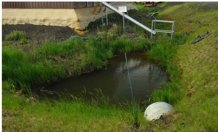
Figure 1: Ineffective culvert due to progressive surface subsidence resulting in constant standing water between the building and the road. The situation is exacerbated by the fact that the local water treatment system continuously discharges water into this pond.
